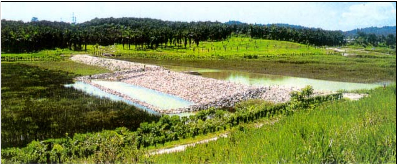
PLATE 1 : A view of wetland cells in the Upper West Wetlands with an extensive planting of macrophytes. Note that the rockfill earth cored weir is used to retain water in the cell.
