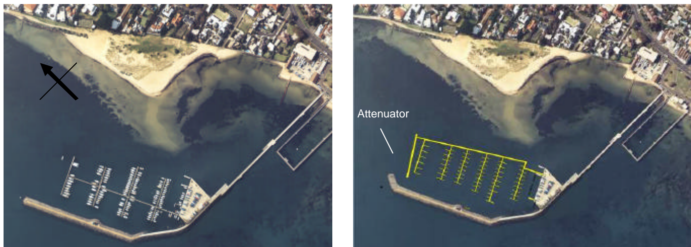
Figure 1. Pre construction marina and simulation of completed marina
