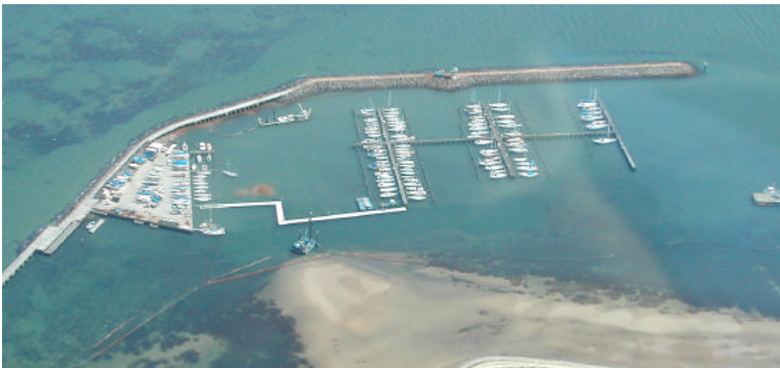
Fig 5 New Marina in progress (pre the floating arms and wave attenuator)
