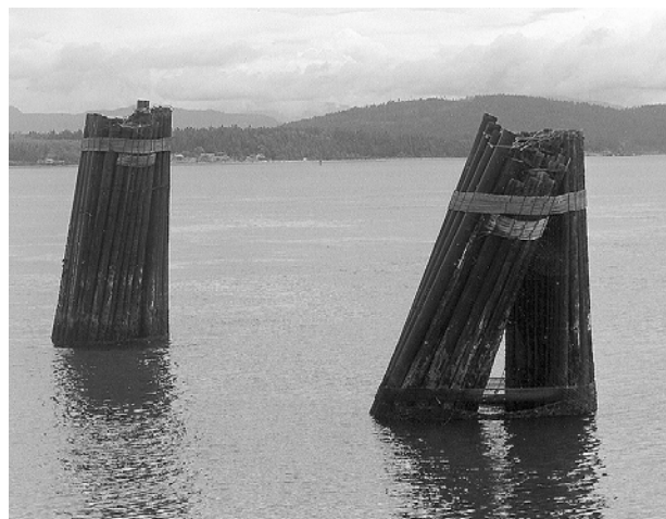
Figure 3: Typical Timber Cluster Pile Dolphins
