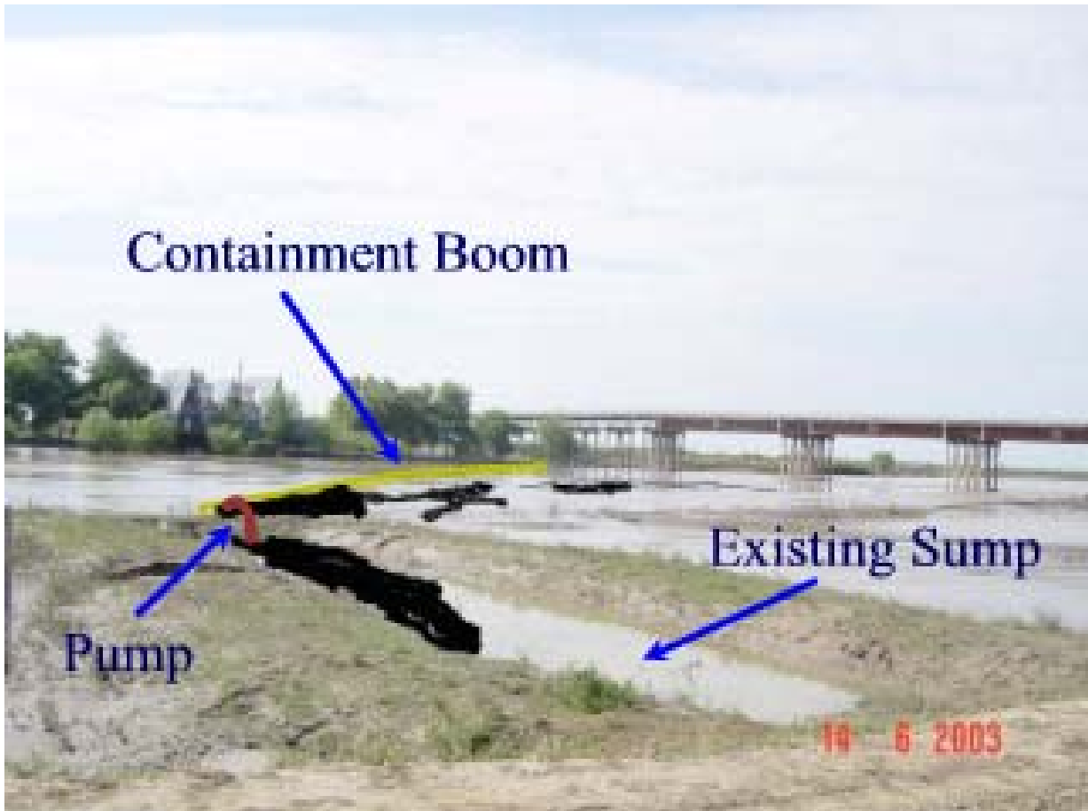
Figure C.1u. Use of Existing Shoreline Sump for Temporary Oil Containment.
