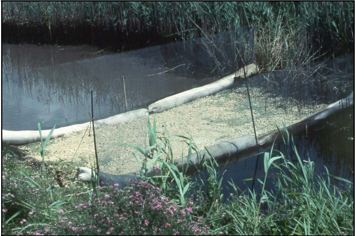
Figure C.4b Filter Fence – Tidal Flow
