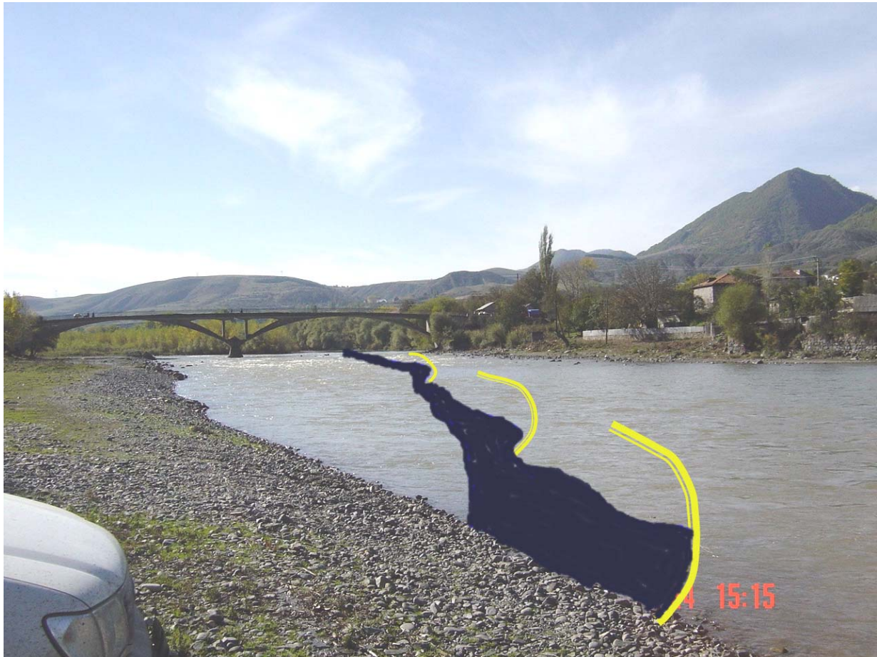
Figure C.1t. Cascading Berms in High Current
