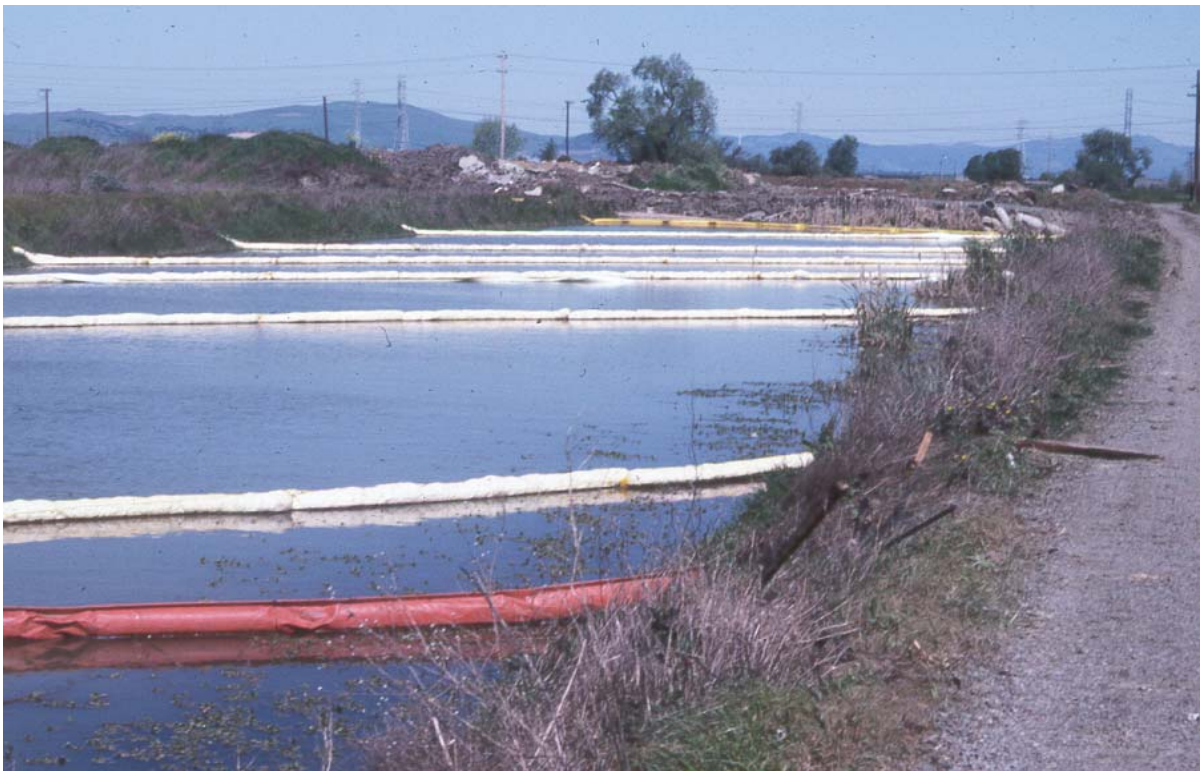
Figure C.1v. Multiple Boom Deployment
