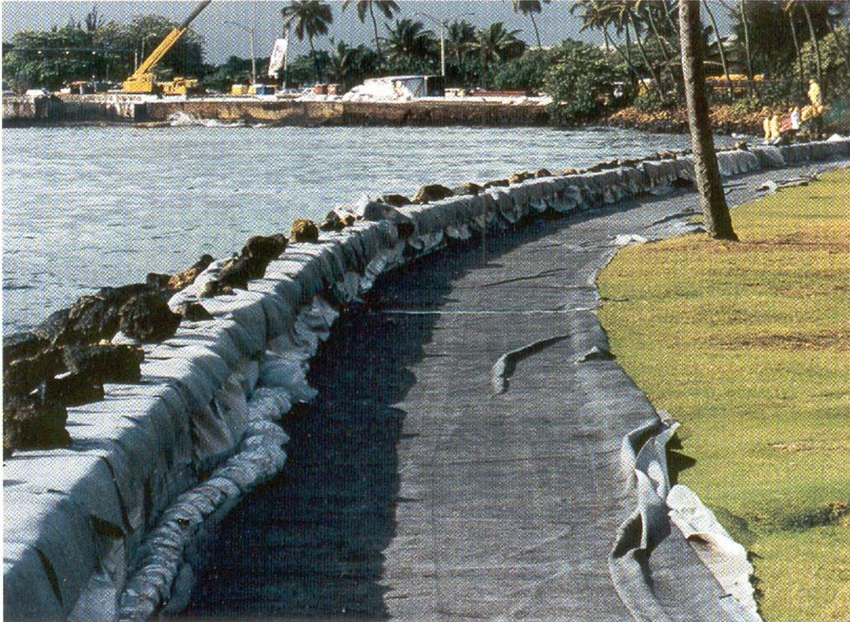
Figure C.3e Shoreline and Backshore Protection
