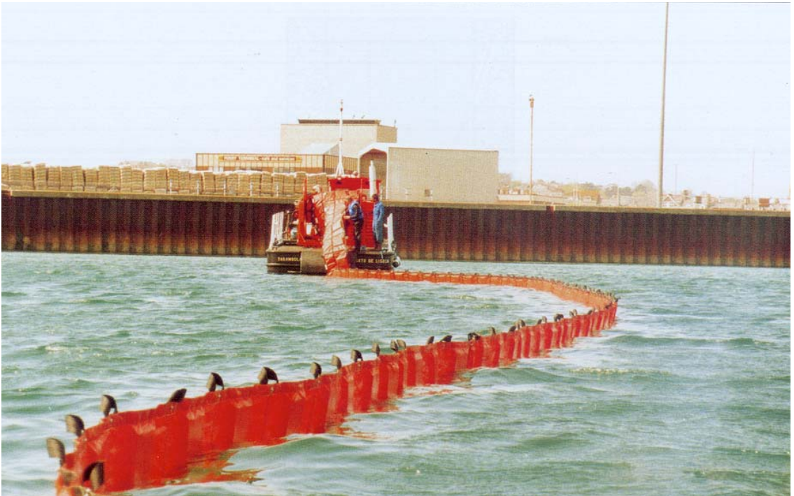
Figure 6 Deployment of a fence boom
