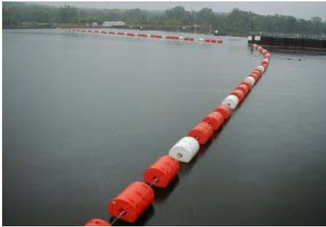
a) Buoyancy boom installation
