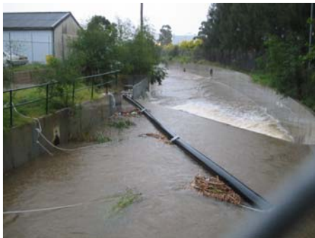
a) Storm Water Drain Channel Installation
