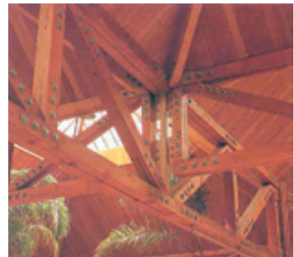
Colour variations between sapwood and heartwood add character to ceiling panelling
