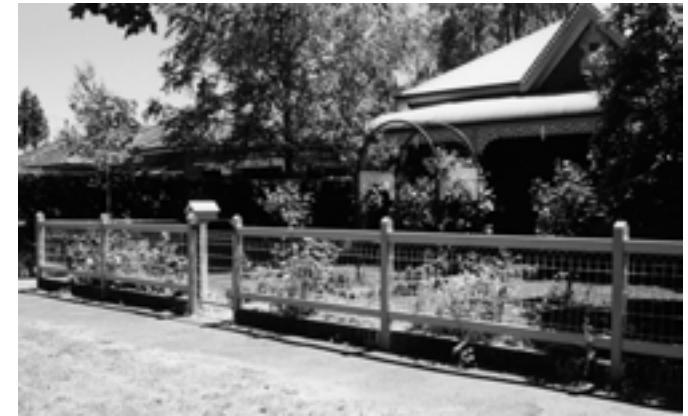
▲ Post and Rail Fence with wire infill
