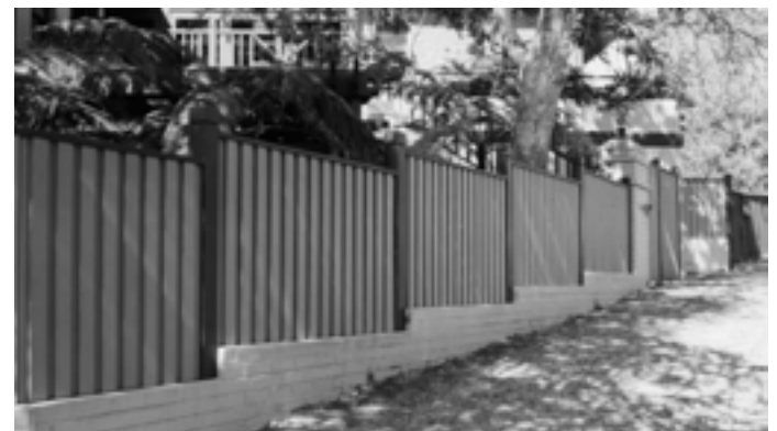
▲ Examples of lapped and capped palings
