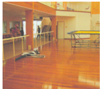
25 mm brush box strip floor designed to take loads up to 5 kPa
