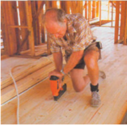
Typical fixing procedure for tongue and groove flooring
