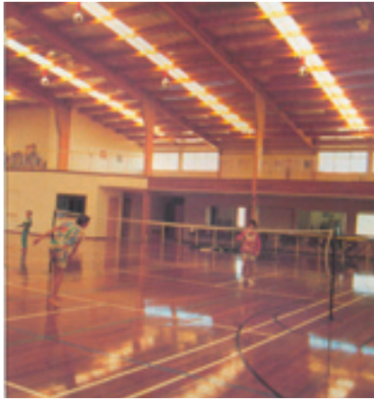
Resilient brush box tongue and grooved timber sports floor
