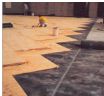
Double layered plywood sheet floor laid over concrete slab
