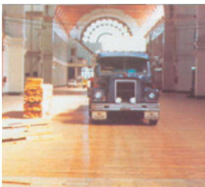
Heavy duty cypress floor designed to take vehicular traffic
