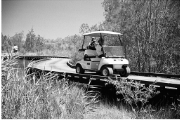
Golf Car Bridge - Owner: Pelican Waters Golf Club
