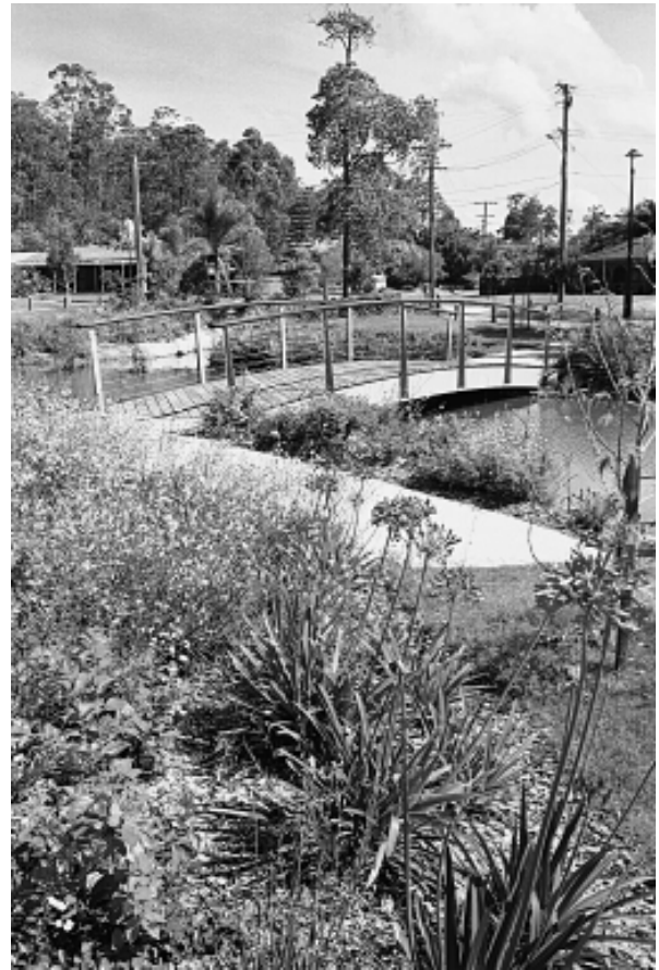
Parallel Flange Channel Girders Bridge - Owner: Logan City Council
