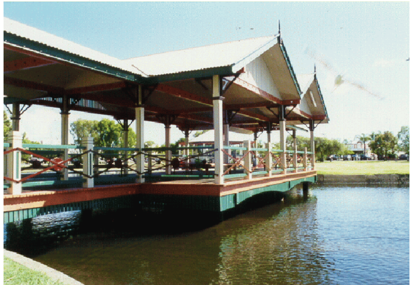
Covered bridge Einbunkin Lagoon, Sandgate - Owner: Brisbane City Council
