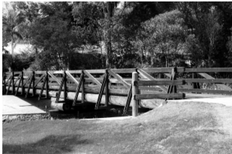
OSA's Log Bridge 2 span with central corbel - Owner: Ipswich City Council
