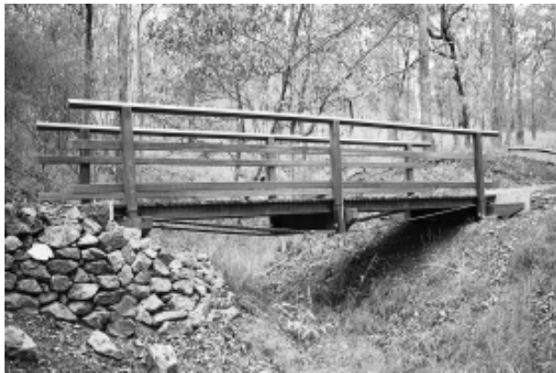
Demountable bridge with 'Barrup' Truss - Owner: Brisbane City Council
