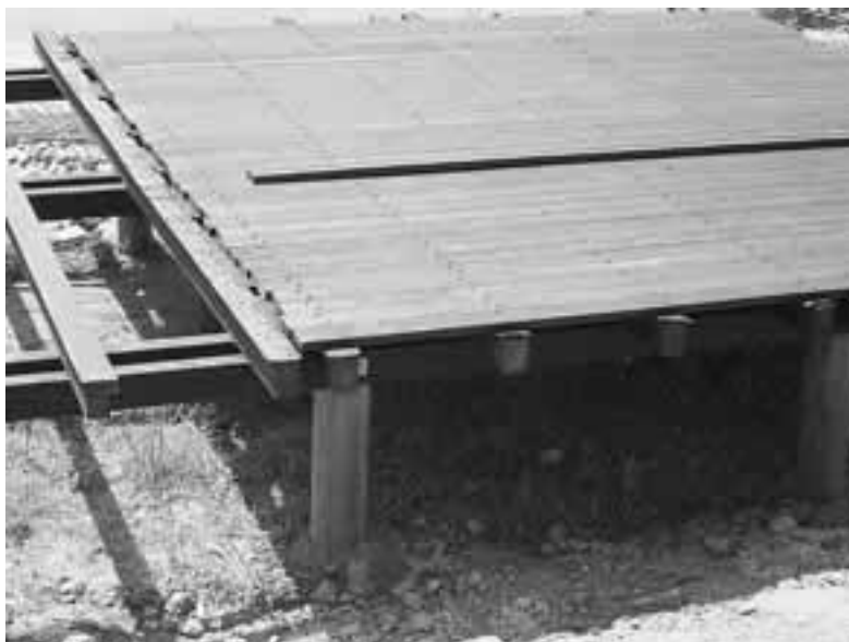
Fig 28 A wide section of deck split into two sections. Note the paired joists. Decking ends are about to be trimmed and a banding plank installed before continuing with the deck.
