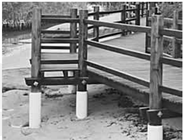
Fig 3 Treated pine piling with UPVC shields in marine
