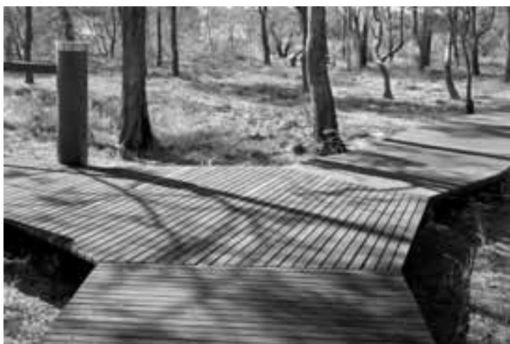
Fig 9 Boardwalk three way junction with truncation
