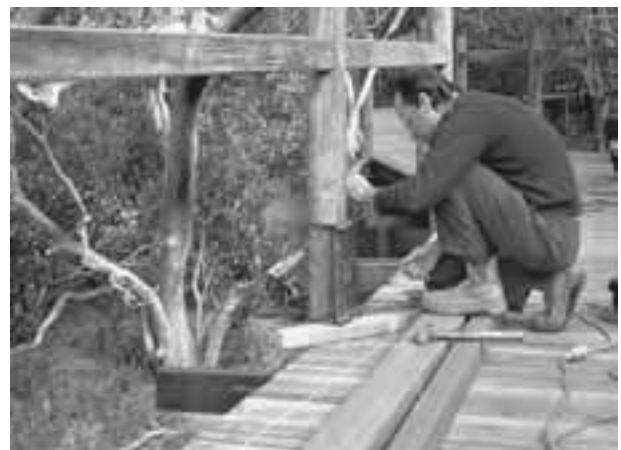
Fig 18 Round handrail post system - router jig
