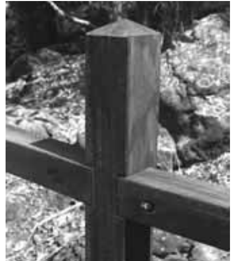
Fig 16 Post projection breaks line of the rail
