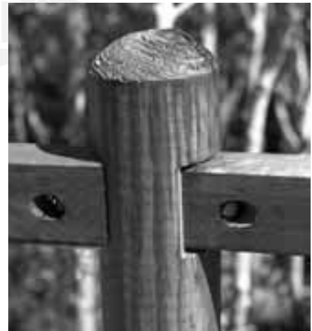
Fig 17 Round handrail post system
