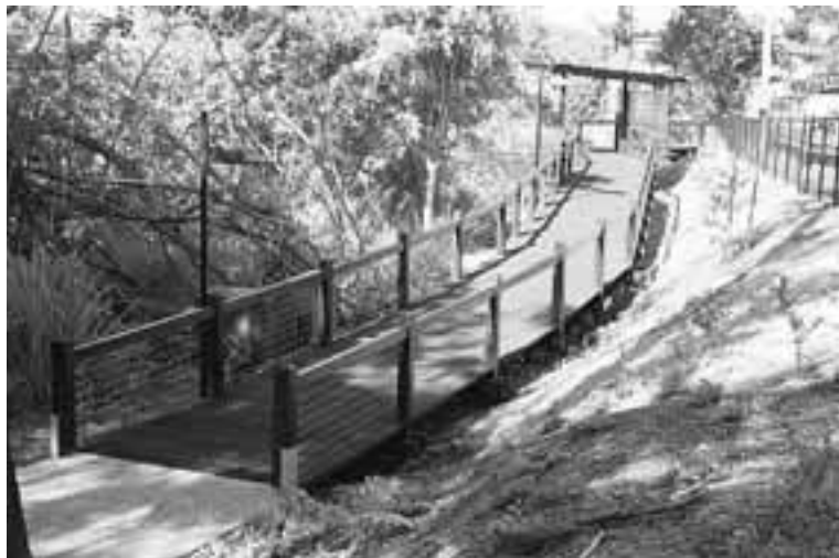
Fig 4. Ramped boardwalk providing access to campus building
