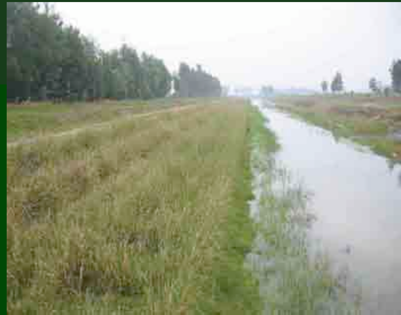
Vietnam - Vetiver stabilizes this irrigation canal
